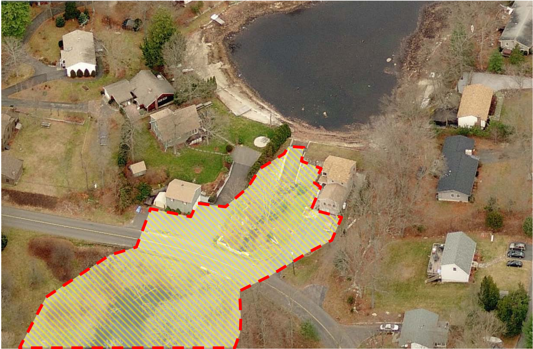
Figure 1 – View of Hidden Lake Dam, looking north and showing the breach inundation area below the spillway and dam.
