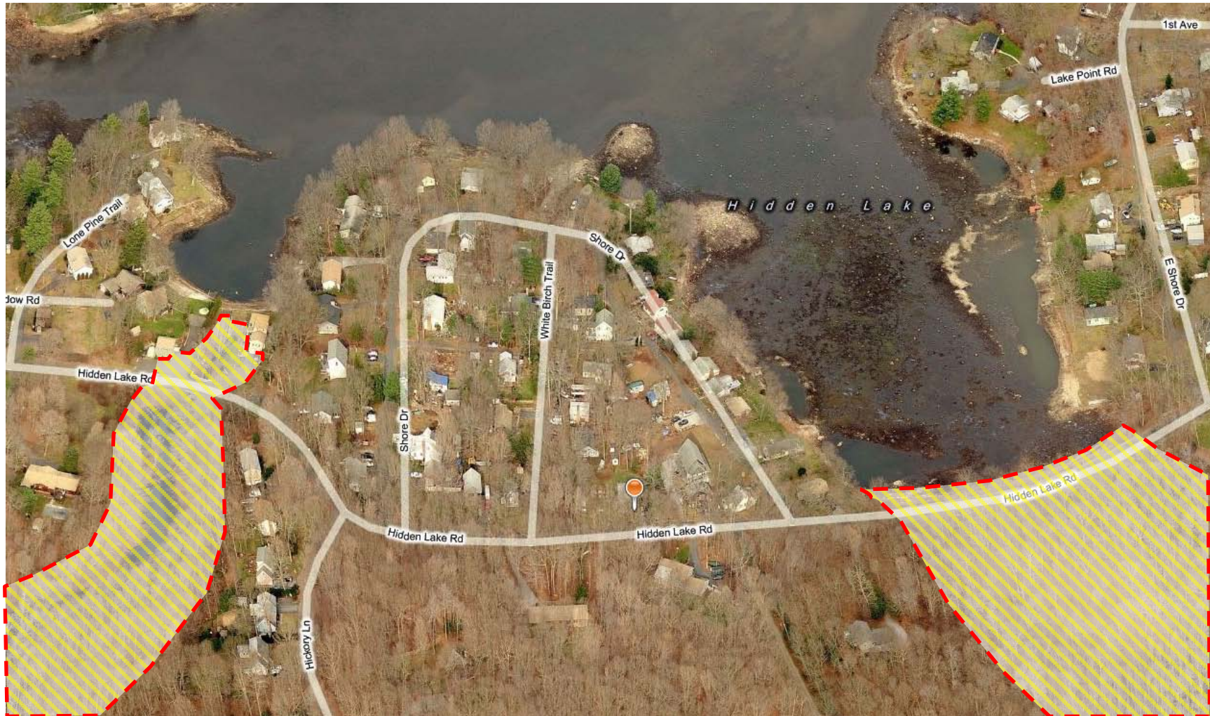
Figure 3 – A view looking northerly toward the pond and showing the breach inundation area on the left and the Hidden Lake Road overflow area to the right. With rising water levels under current conditions, the houses between these two points could potentially be isolated due to road overflow.
